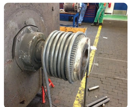
Heating a coupling for dismounting
